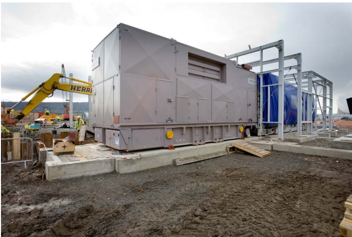
Construction work underway on site of new gas turbine
